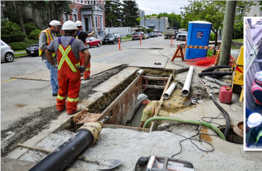
Typical pipe bursting setup
