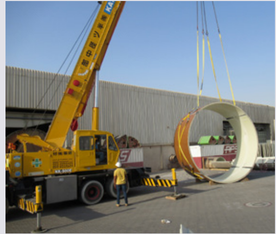
Glass Reinforced Plastic (GRP) segments are becoming more widely used for sliplining
